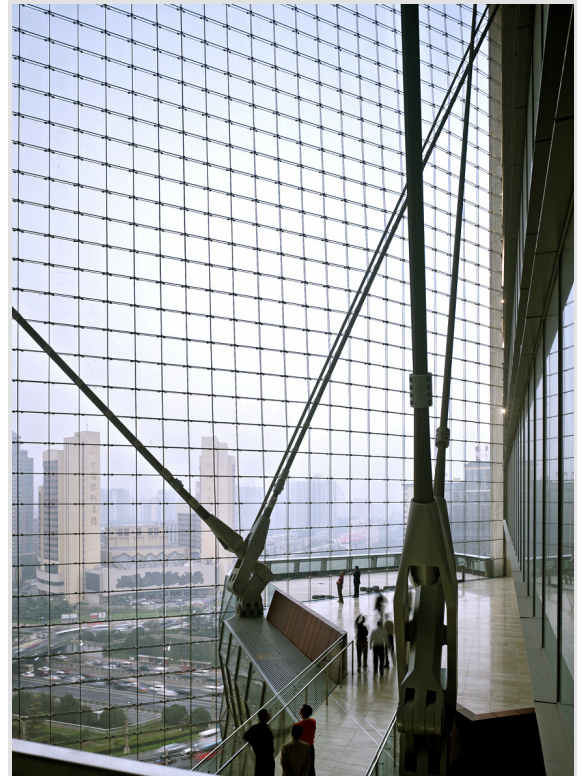
Figure 2: Main cable-net wall with primary 'v cables' (Photo: Tim Griffiths, Skidmore, Owings & Merrill LLP)
