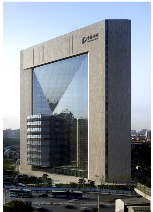
Figure 1: Beijing Poly Plaza (Photo: Tim Griffiths, Skidmore, Owings & Merrill LLP)
